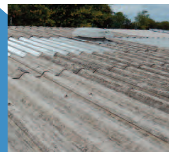
Cleaned Roof Surface
