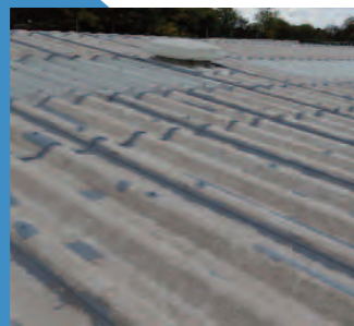
Liquasil Non-Sag Sealer to Overlaps and Cracks
