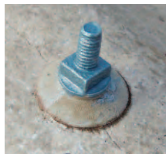
Metal fixings treated with Liquasil Corrosion Primer
