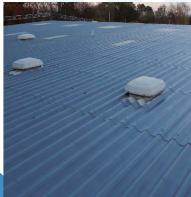
Asbestoseal 20 to entire Roof
